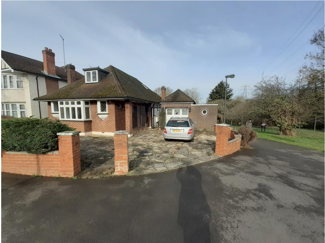
Site property is a corner plot with a detached bungalow. Yeading Walk to the northeast.
