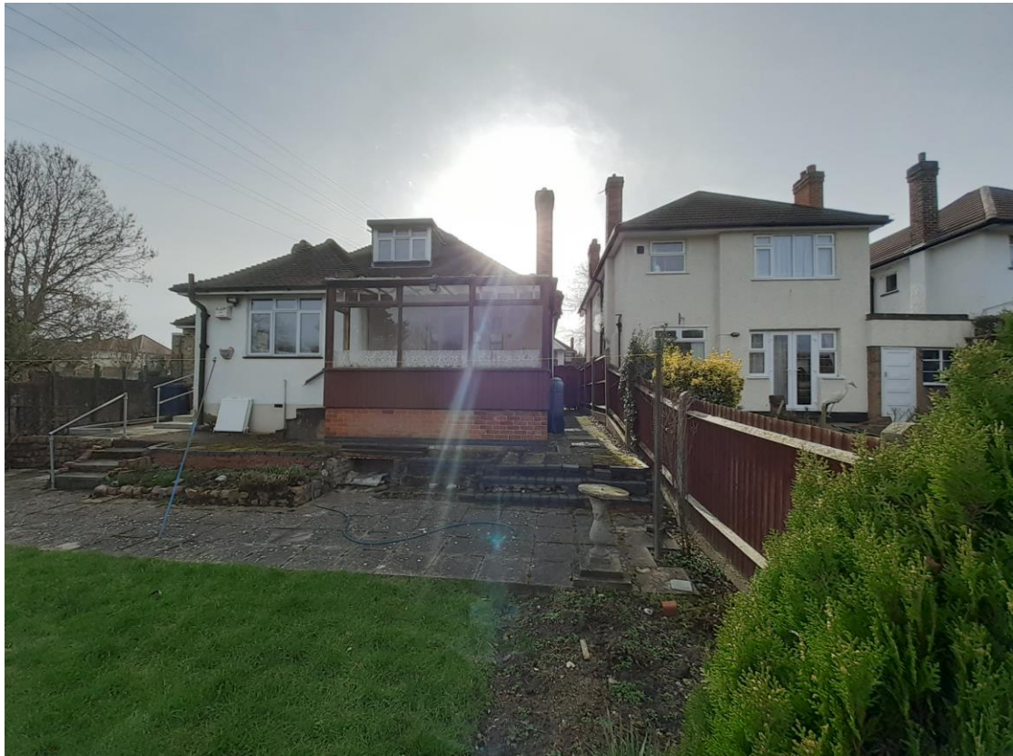
Rear view. Existing conservatory (centre). No.44 (right)
